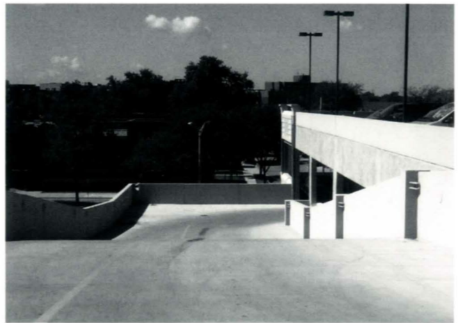
While installing ramp No. 3, the contractor spaced the cable tighter than designed and ran out of cable before fully covering the area to be heated. Delta-Therm supplied an extra cable, and a spare circuit in the contactor panel accommodated the extra load.
